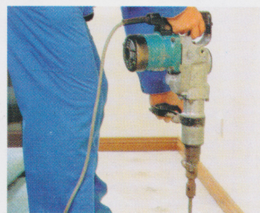
Concrete slabs have to be drilled.
