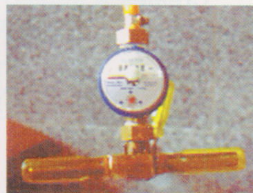
Each hole is filled with 5 liters solution.
