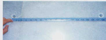
Holes are drilled at a distance of 50 cm.
